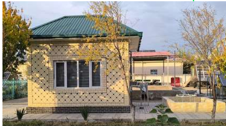
Figure 2. General view of the experimental house
